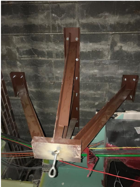
Structural Steel for Swing
